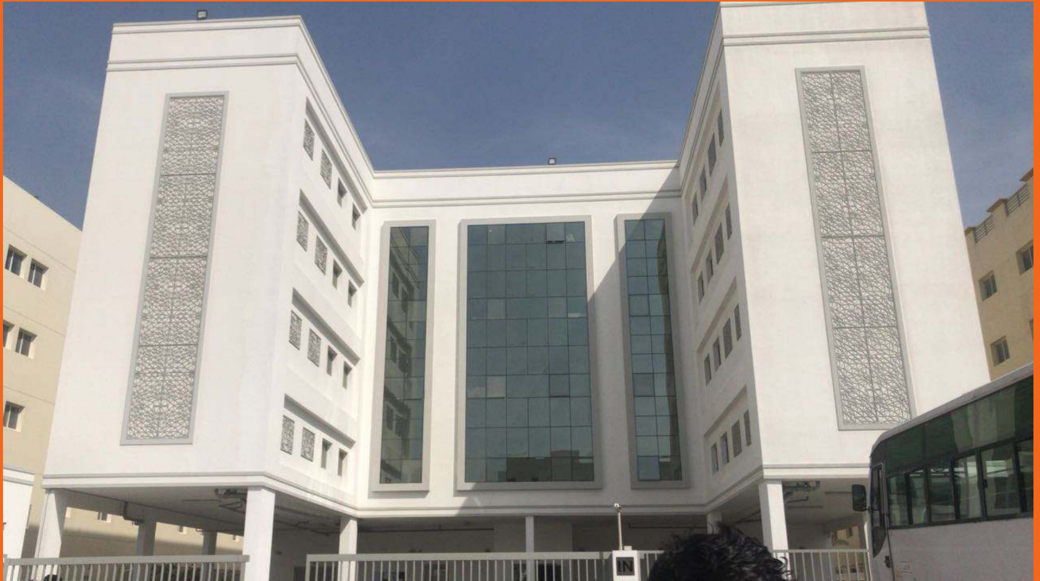
(Gr+4) Labour Camp Accommodation, DIP, Dubai | Client : M/s. Prestige Constructions LLC
